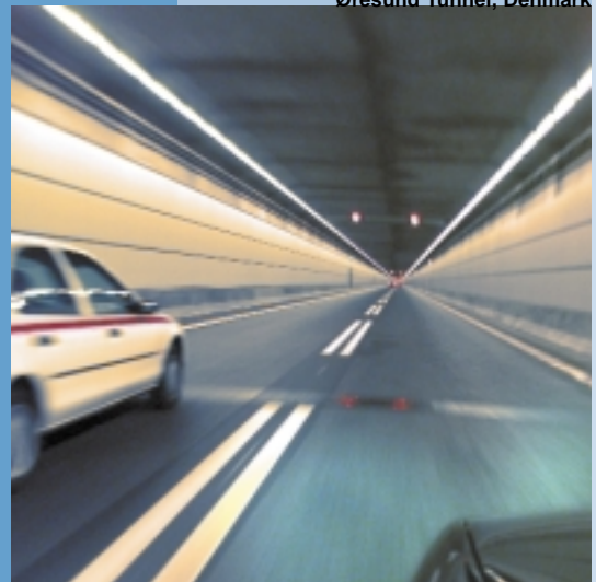
Øresund Tunnel, Denmark
