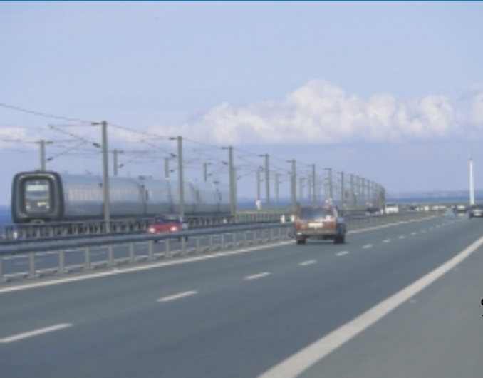
Great Belt West Bridge, Denmark
